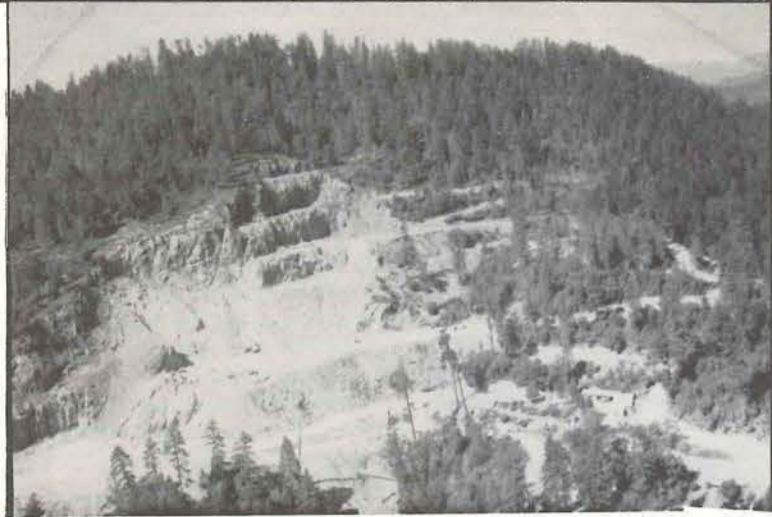
IDEAL CEMENT company's quarry at Wilderville, Oregon.
