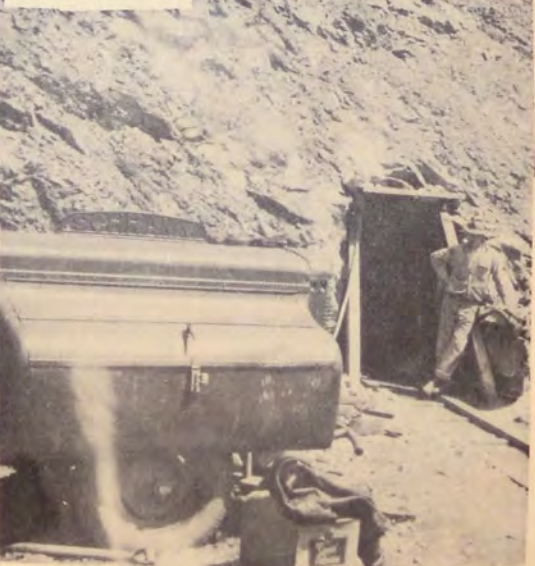
FRED LANGLEY AND CLAUDE DEAN, GRANTS PASS, OREGON, HAVE BEEN OPERATING THE BIG BEAR PROPERTY SINCE JUNE, 1952. IT IS ABOUT SIX MILES UP SLATE CREEK FROM THE REDWOOD HIGHWAY. A CROSSCUT, 75 FEET LOWER IN ELEVATION THAN THE ORIGINAL WORKINGS HAS BEEN DRIVEN. MORE THAN 200 TONS OF CHROMITE HAVE BEEN MINED FROM THE ORIGINAL ADIT AND STOPE, AND A CHROMITE LENS WITH A MAXIMUM WIDTH OF ABOUT 7 FEET IS EXPOSED IN THE FLOOR OF THESE WORKINGS. ON MAY 4, 1953, ORE WAS FOUND AT 310 FEET.
