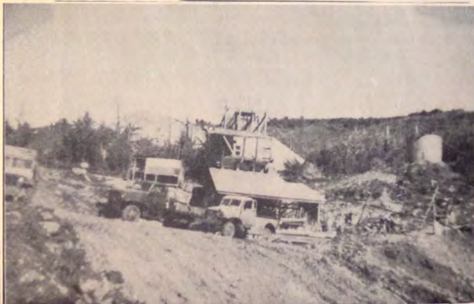
INTERNATIONAL METALLURGICAL CHROME CORPORATION MILL OPERATED BY H & J CHROME CO. LOCATED ABOUT 9 MILES WEST OF SAN LUIS OBISPO, NEAR THEIR MINING PROPERTY. CAPACITY OF MILL IS 200 TONS OF HIGH GRADE CONCENTRATES PER DAY. RAIL SHIPMENT MADE FROM GOLDTREE SIDING ABOUT 8 MILES FROM MILL.
