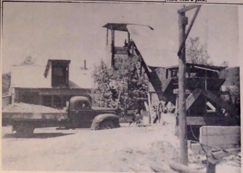
LYTELL MILL ON HIGHWAY 40 WEST OF AUBURN, CALIFORNIA
