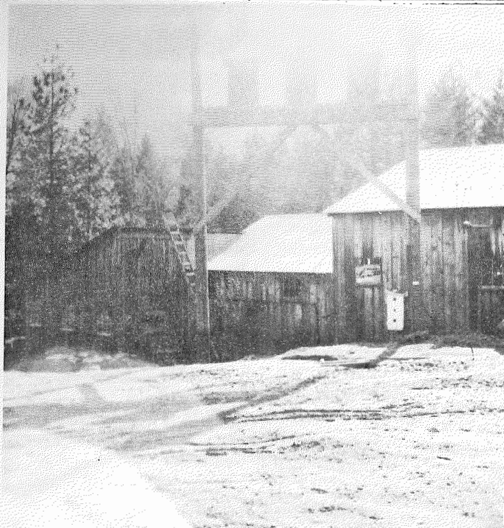
LOWER PART OF BUILDING, CASTELLA MILL.
