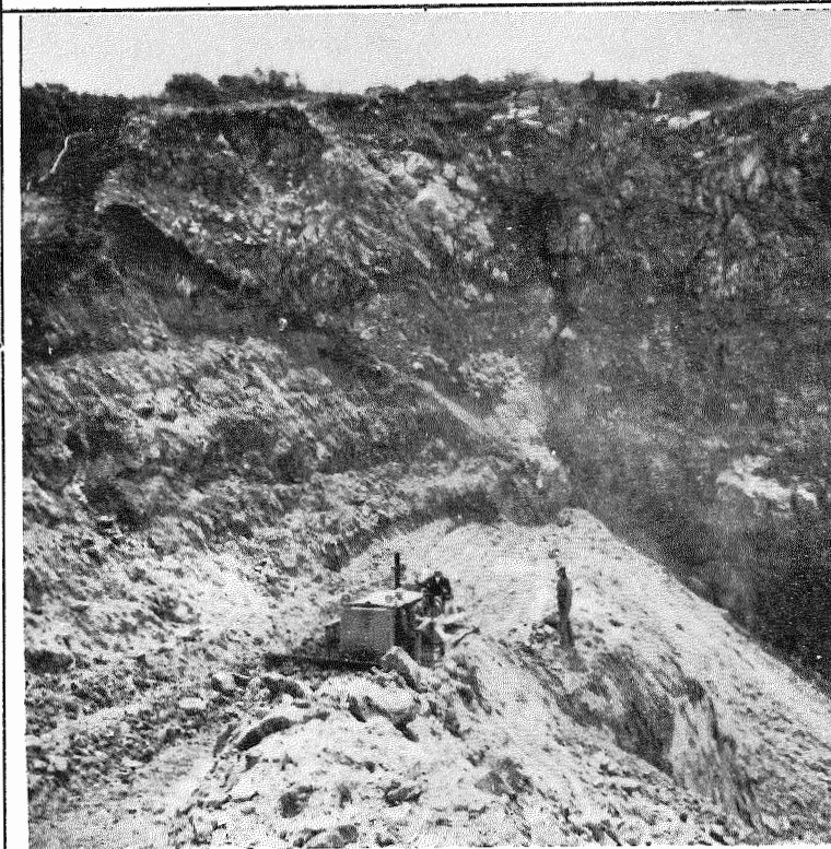
CASTRO MINE. D8 stripping new ore body. East pit.
