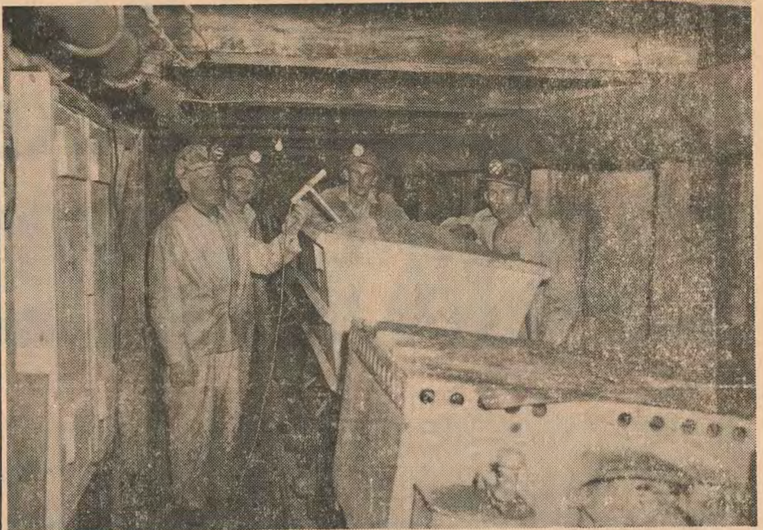
Most White King ore for the uranium reduction plant has, until recently, come from underground. This group of miners is shown checking a carload of ore, at the 6130 station, for radioactivity to check its content of uranium oxide. A recent change
