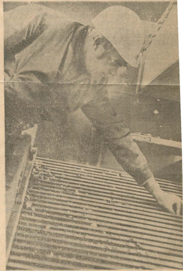
PICKING NUGGETS — Cornucopia President Howard Yates "high-grades" the sluice box he had fabricated in Seattle for the Pine Creek mine. Riffles the under-laid with carpeting, which catches fine gold.
