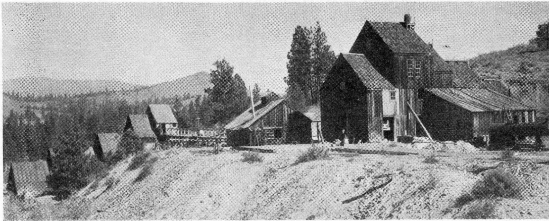
Gem of Sparta mine buildings at the right. The collar of the old shaft is inside the building. The new shaft inclines into the hill behind. The mill buildings are at the left of the picture.
