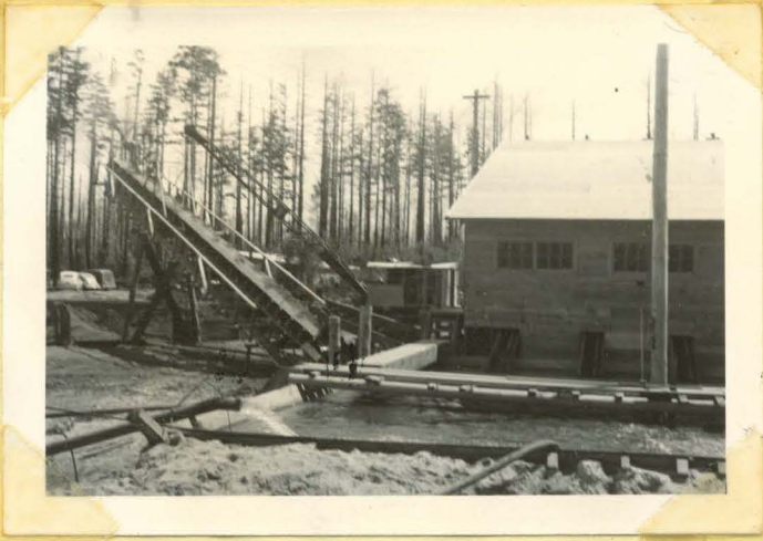
Concentrator: looking N.E.
