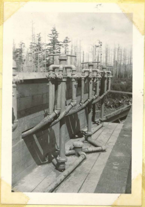
"Christmas Tree" valves delivering sand to Concentrator.
