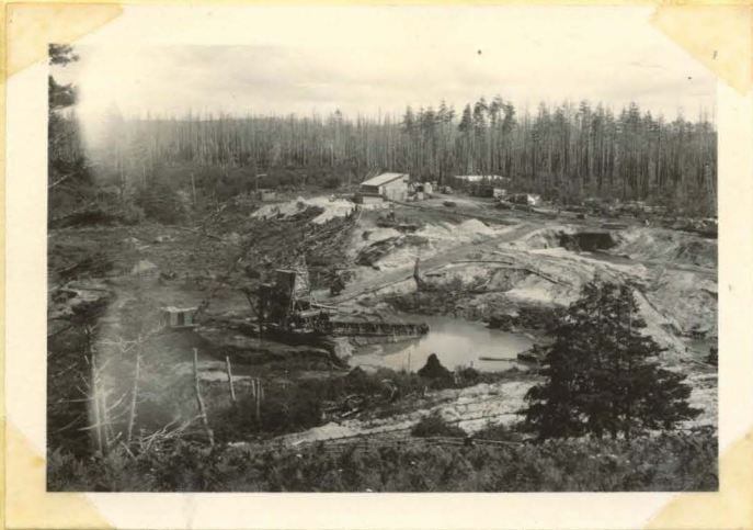
General view looking south across the Lagoon. Washing plant in middle foreground. Concentrator in background. Sand is pumped up to Concentrator.
