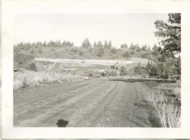
Close-up showing Williamson pit and crushing plant.
