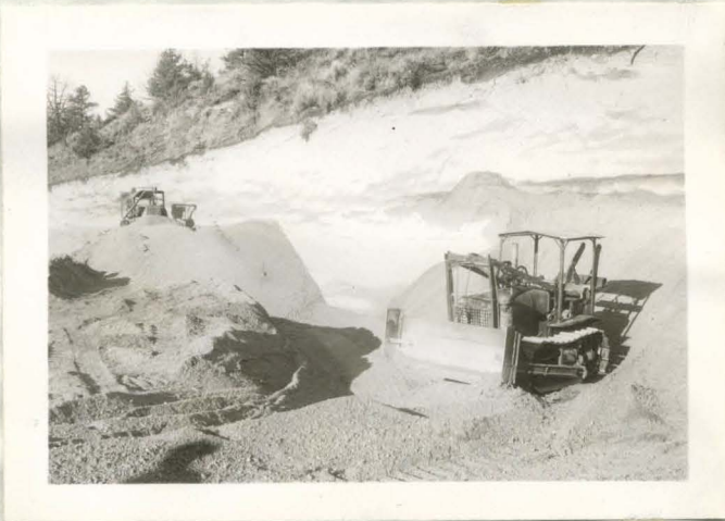
View of Williamson pit from feed chute of plant. The extremely white area on the lower half of the face in the center of the picture is the pumice in place. When dozed loose it assumes the color of the piles in the foreground. Pink ash overburden extends from grass root level down to the top of the pumice.
