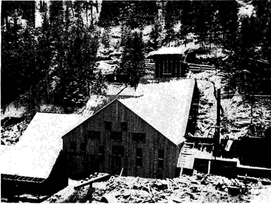
New mill of Cougar-Independence Lessees at Granite, Ore. Portal of new tunnel being driven to cut veins of both mines at lower level is behind first trees to the left of the ore bin.
