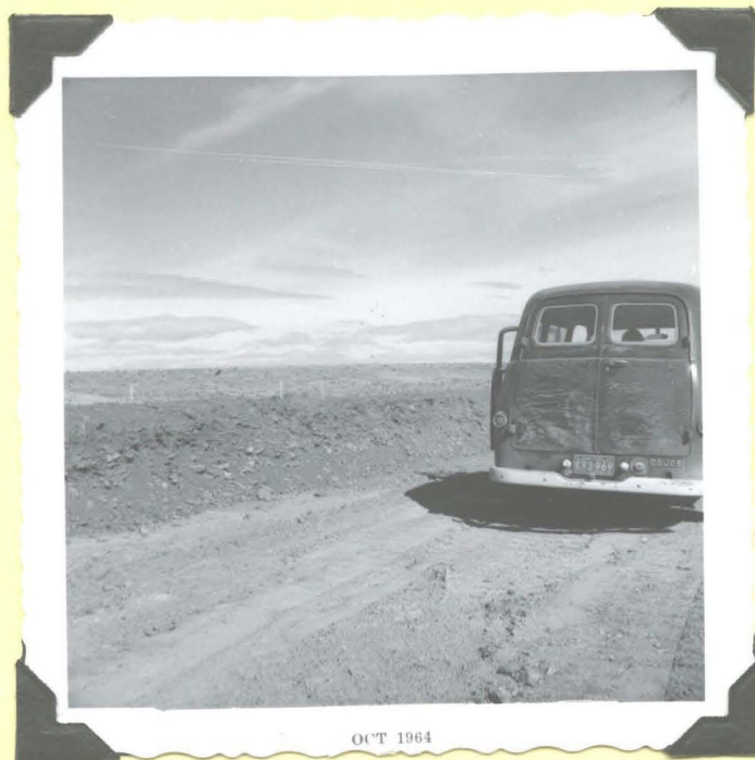
View northwestward from one of the streets in the subdivision. Shown is the rock-soil nature of the material being excavated.
