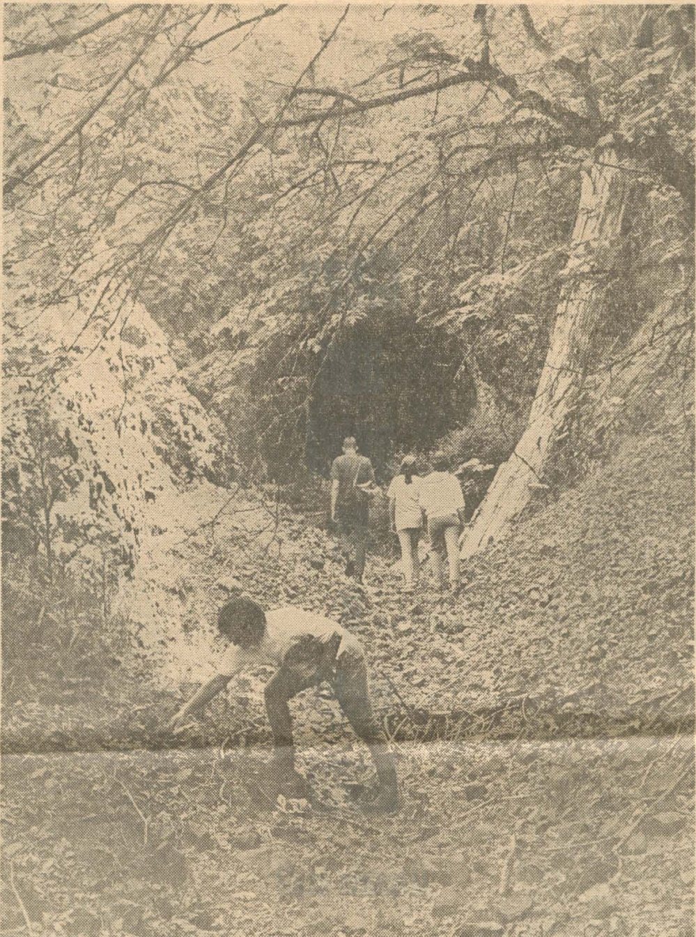
GLOOMY MOUTH of abandoned Buck Rock Tunnel near Ashland looms before trio bent on exploring the famed tunnel. Old O&C Railroad Company started what would
