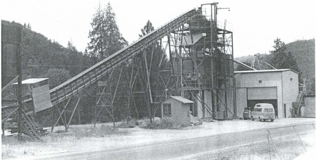
Figure 5. A portion of the Bristol Silica and Limestone Company processing plant where crushed quartz from the pit is further crushed, screened, and bagged.
