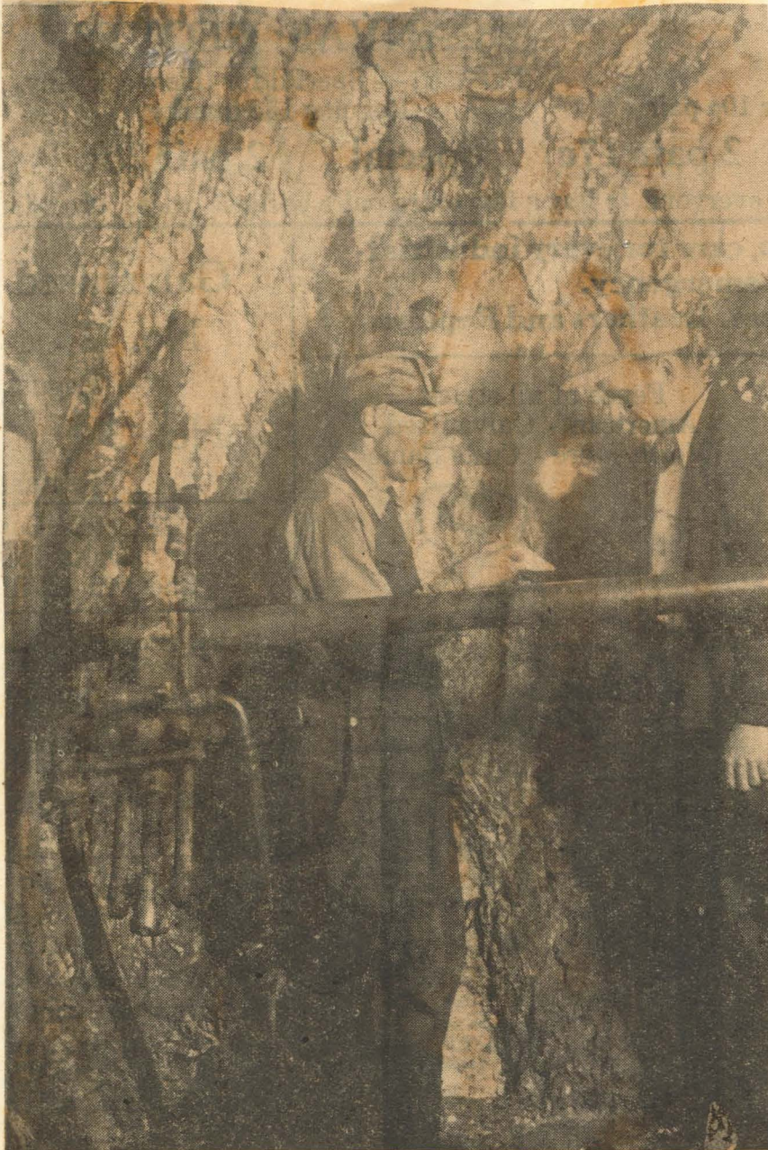
Miners with air drill one of the tunnels at the Oriole mine, one of the important quartz properties in the Galice district. The mine is owned by Harry Sordy and is being operated under a lease by Charles Benson and Ben Thomas. Several thousand dollars have been spent during the past year in new equipment.
