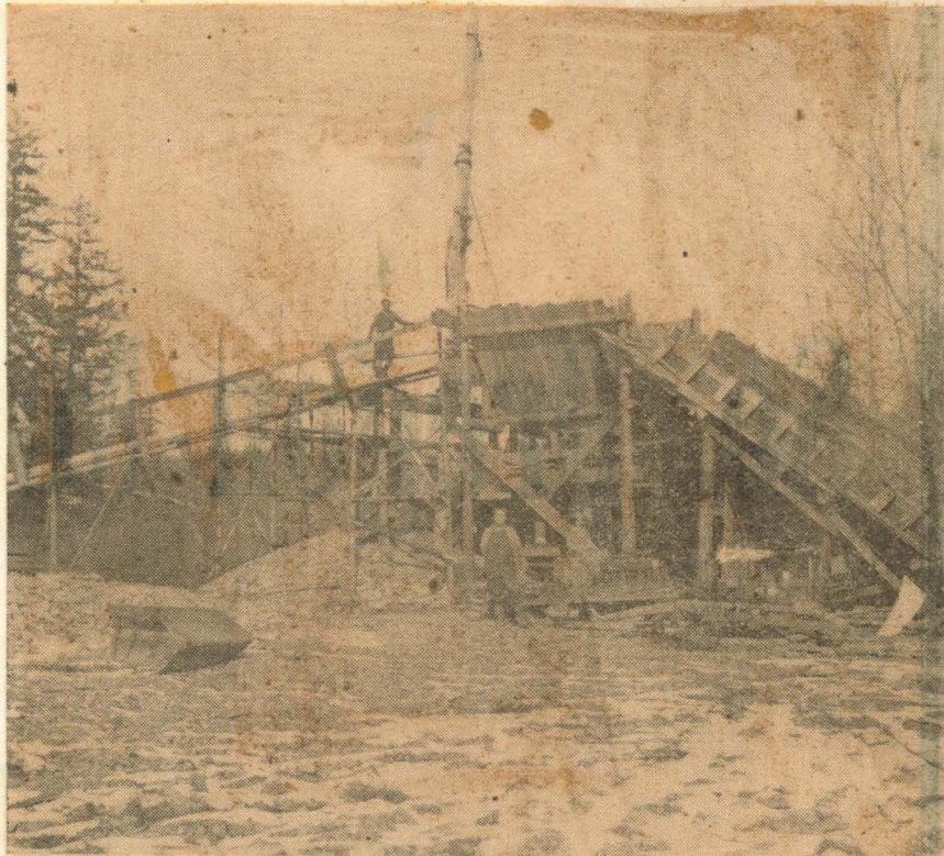
Chinese mining operations may still be found in Josephine county. Wong You and his two sons are getting ready to resume operations on the Rogue river near Finley Bend. Photo shows hopper to which Wong hoists the material, the hoist being operated by an old Packard engine. A smaller engine pumps water from the river, the gravel is washed and passes into the sluice on other side of hopper where a series of different types of riffles extract the fines. Wong's eldest son is shown on top of the elevated hopper. Wong himself below.
