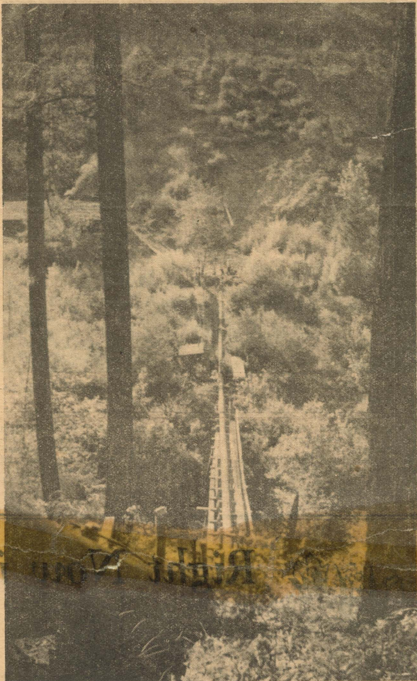
View of Elkhorn mine, old-time heavy producer, showing part of pipe-line laid through rugged Briggs Creek section of Josephine county. The mine is now ready to operate again after a year and a half of construction work, including new flumes, ditches, roads and pipe lines to carry water for hydraulicking.
