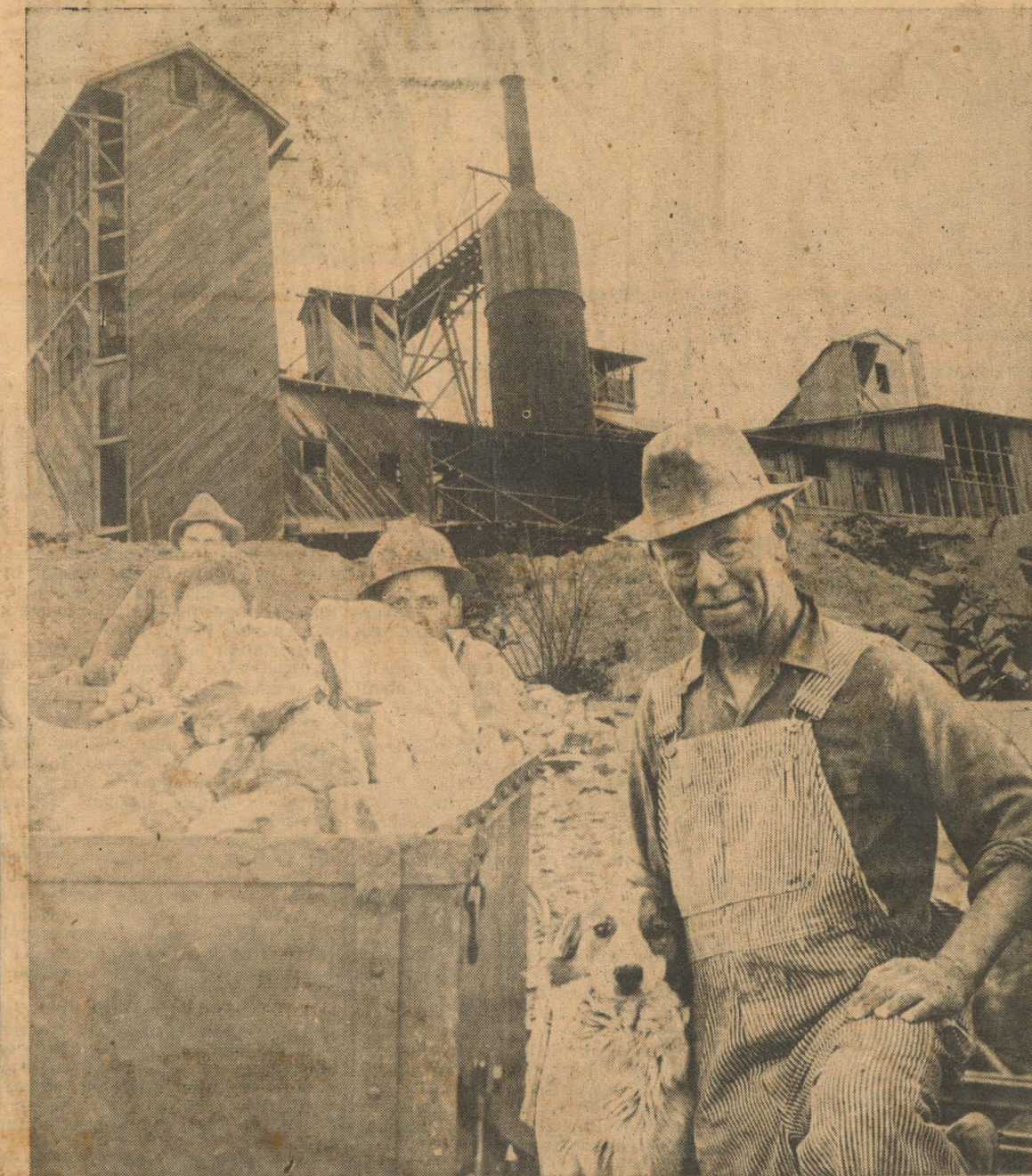
The test of fire has been applied to Josephine county limestone, and it has proved satisfactory for exacting requirements of industry. Above is shown part of the plant near Williams and Provolt. The quarry is directly behind the structure, while the dumps in front of the plant obscure the entire lower story of operations. The kiln, operated by V. Z. McCary, pictured at the right with his dog Pat, is the only one operating in the state. On the left, raw limestone is shoveled in mine cars from quarry to kiln. About 15 local men are regularly employed. (Courier Photos and Engraving.)
