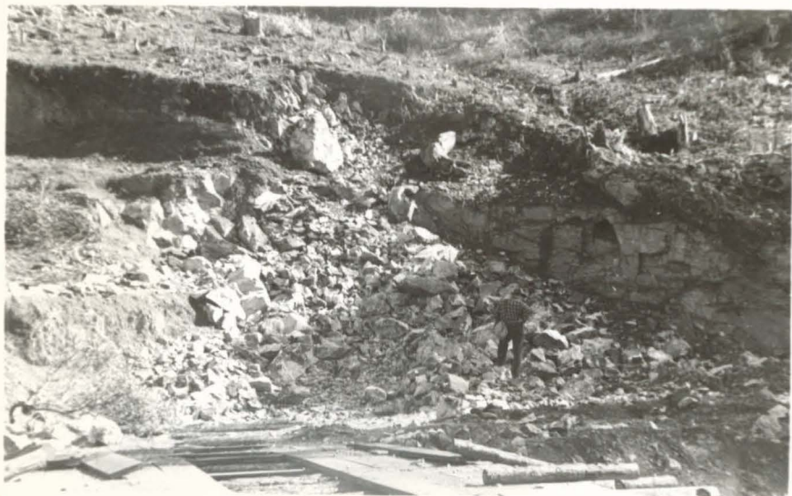
Debris at lower quarry in front of slope.
