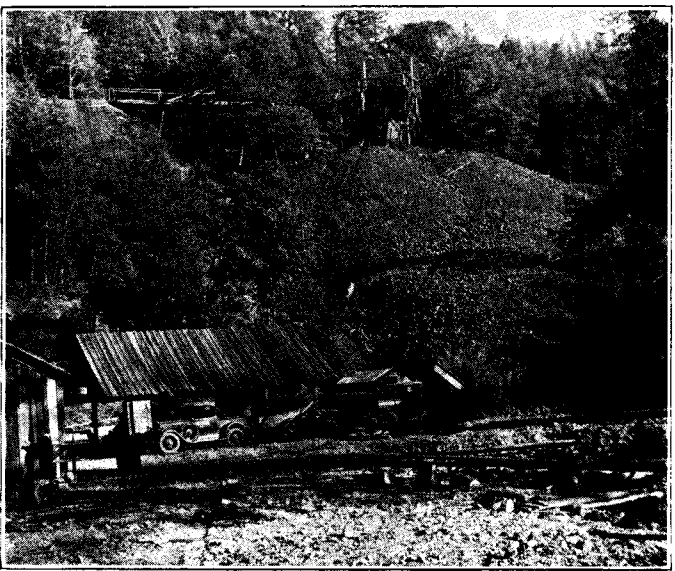
QUEEN MINE—Showing Sulphide Ore Dumps
