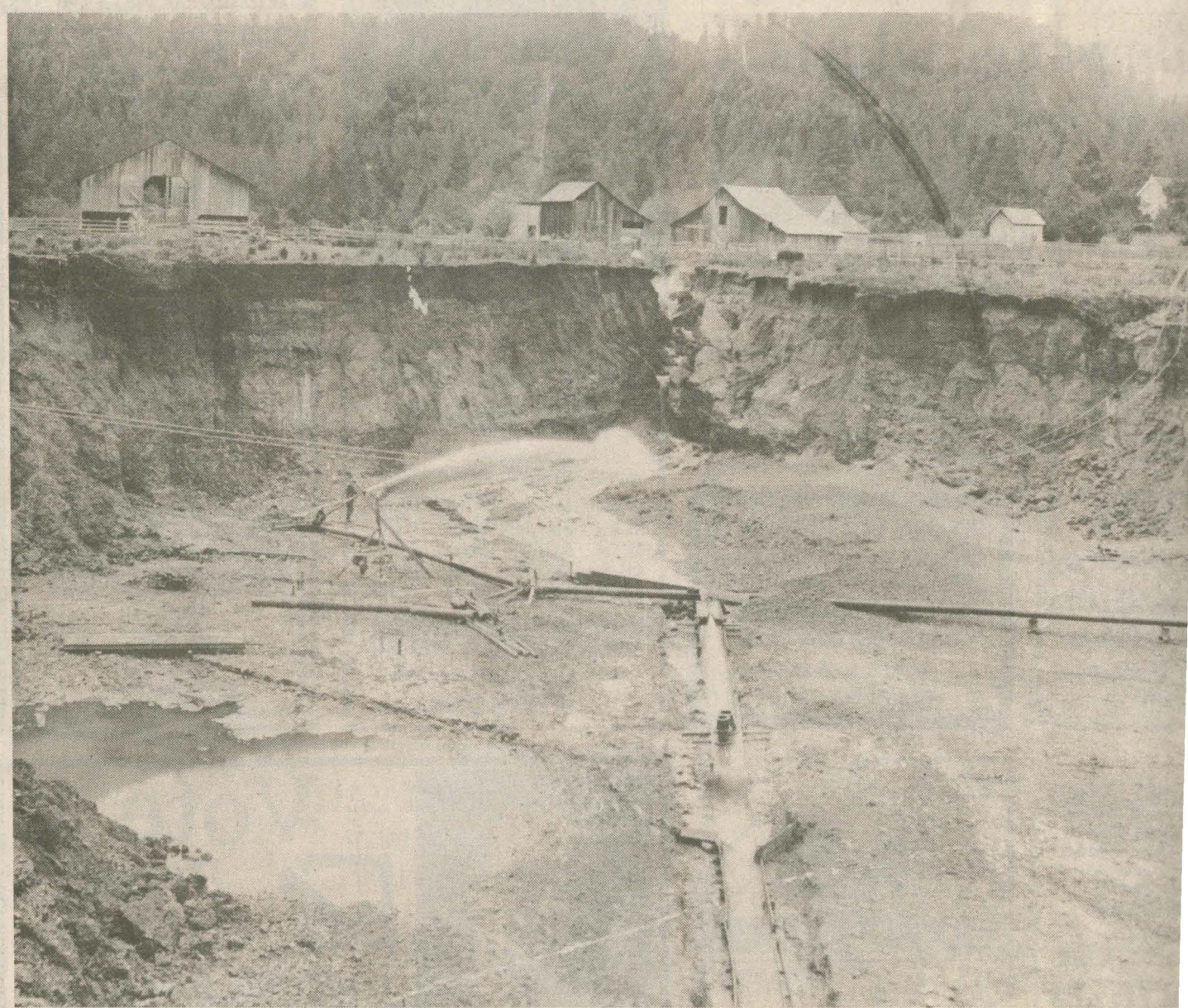
HUGE MINE PITS, dug by hydraulic nozzles called "giants" Logan mine. A ravine was dug to the north of the p arved down into a cow pasture to create the Simmons, Cameron, water to the east fork of the Illinois River. This pho
