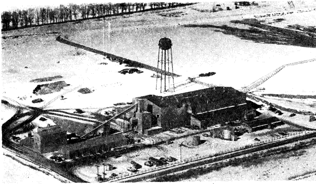
GENERAL view of the uranium reduction plant at Gunnison, Colo., where the Gunnison Mining Company processes ore from its leased Los Ochos mine. That company is owned by the same group of partners who own the Lakeview Mining Company. (Western State Aviation photo by Rocky Warren, Gunnison, Colo.)
