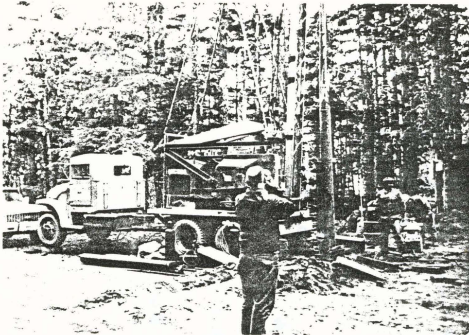
Slide 5a, Northwest Natural Gas Company's Drilling at Old Maid Flat
