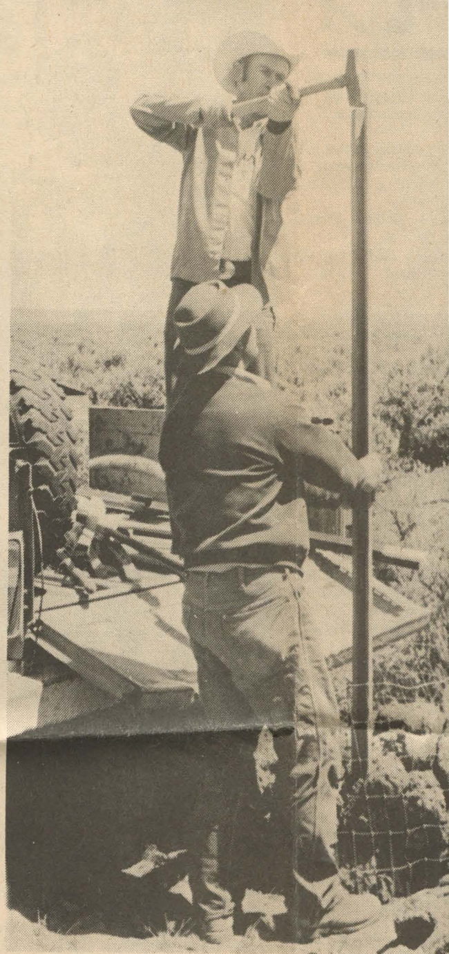
STEEL POSTS protected by rock bases were used for the boundary of the sunstone reserve.
