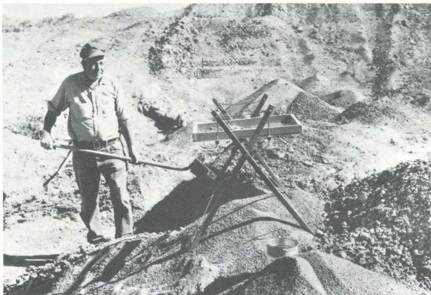
Figure 10. A typical sunstone mining operation. The thin overburden has been removed exposing decomposed basalt, which is easily disintegrated by hand picks and chisels and then screened to separate the sunstones.
