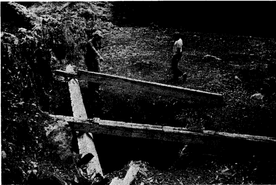
Figure 11. Part of old Musick mine workings which have reached the surface (checkpoint 36). Shafts like these are very dangerous, so stay away from them.
