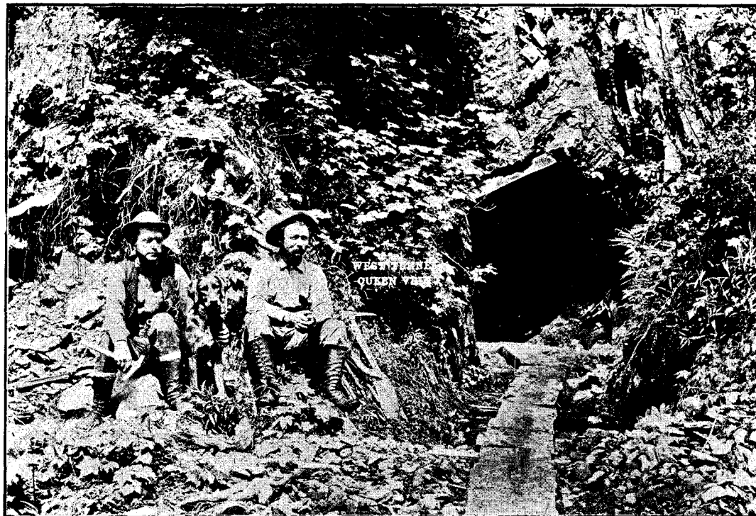
West Prospect Tunnel on Queen Vein. The face of this tunnel is 300 feet from face of East Tunnel, all showing ore-bearing formation.
