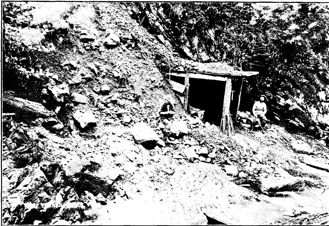
East Prospect Tunnel on Queen Vein, showing ore formation, width from hanging wall to foot wall about 130 feet.
