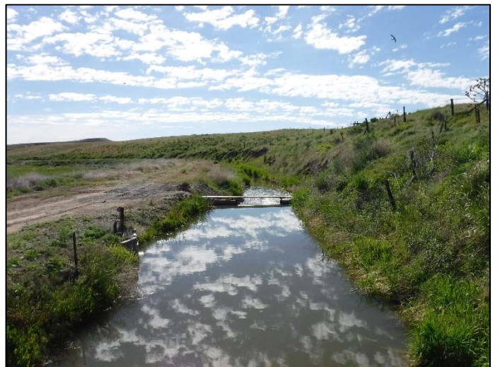
J-H Canal (artificial waterbody) facing downstream. Berm is visible on right bank, and water control structure is visible on the left bank.
