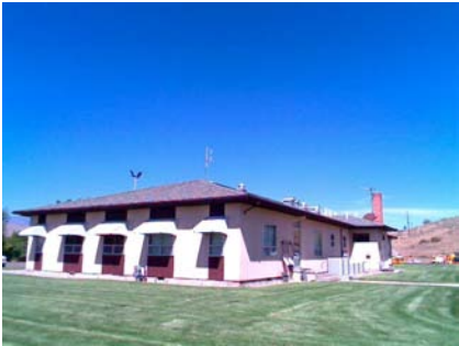
SE Secondary Structural Type
