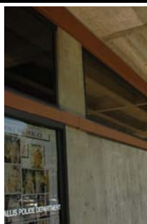
S Vertical Irregularity Secondary short column
