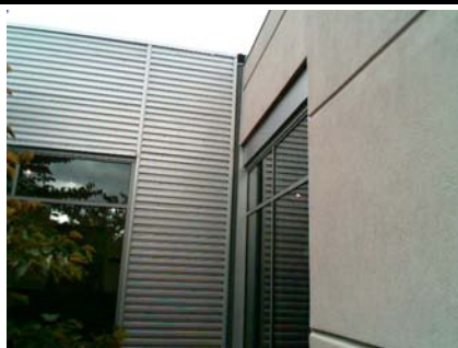
S Seismic Upgrade 3" SEIS JT
