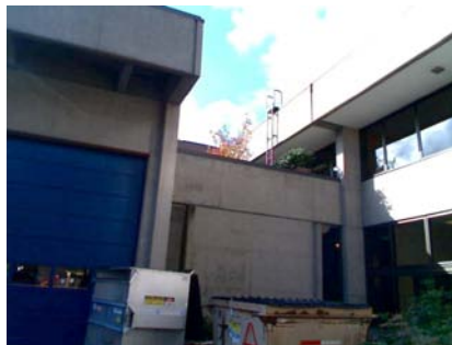
N Vertical Irregularity Primary CONN OF S WING AND CENTER
