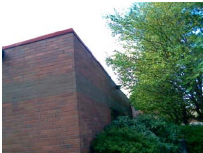
NE Elevation View
