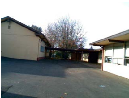
E Pounding Potential a on left, b on rt. Pounding on a only.
