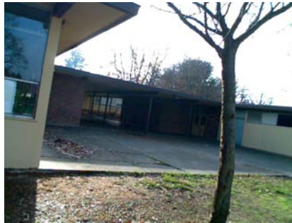
N Plan Irregularity Primary breezeway between e and w wings
