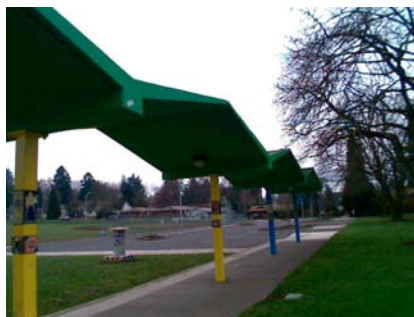
N Falling Hazard conc canopy
