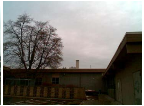
W Falling Hazard old cmu chimney looks unreinf
