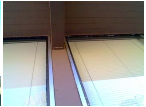
E Plan Irregularity Tertiary LOOKS LIKE CONN MAY HAVE BEEN DESIGNED TO HOLD SOME LATERAL FORCE WITH PLATES SURROUNDING BEAM. SHO
