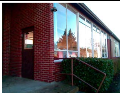
N Plan Irregularity Primary can see through to outside wall beyond, with also large window areas
