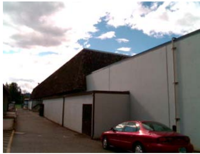
SE Secondary Structural Type PC, RM AND C2 SECTIONS VISIBLE
