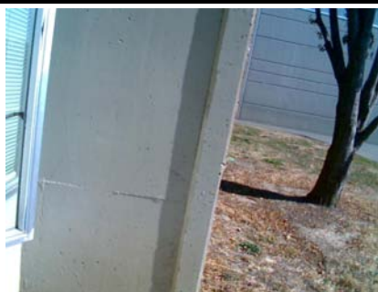
S Primary Structural Type FORM MARKS, NO CAULKED JTS
