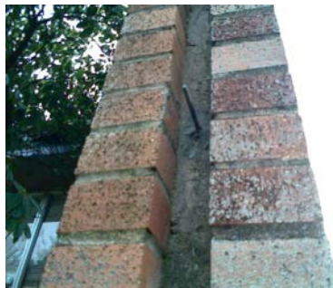
N Secondary Structural Type cavity wall
