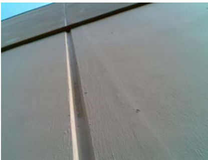
S Primary Structural Type caulked vert jts and cladding
