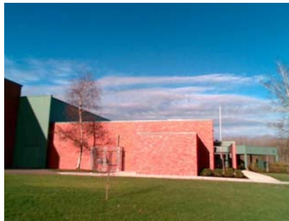
S Vertical Irregularity Secondary note free-standing brick wall - 12" thick
