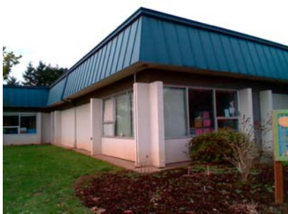
N Primary Structural Type
