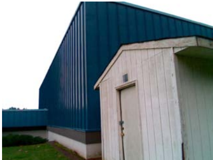
SE Secondary Structural Type
