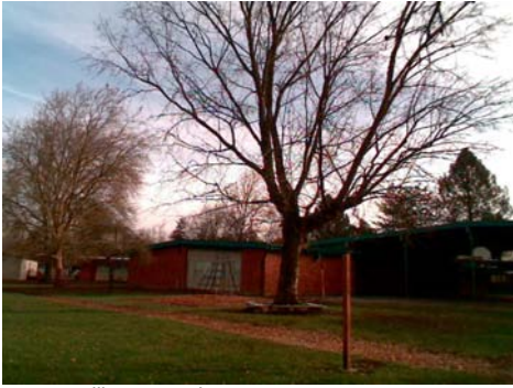
NW Falling Hazard part 3 and 4
