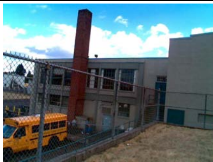
N Falling Hazard
