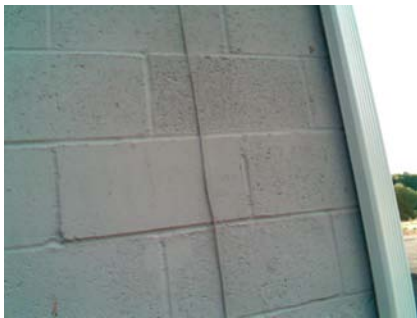
SW Primary Structural Type
