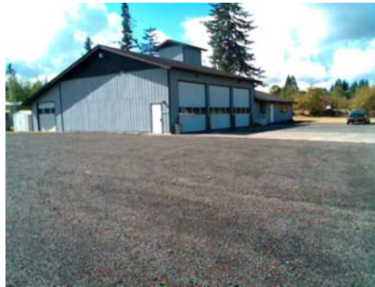
NE General Site
