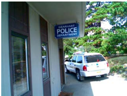
SE Building Name
