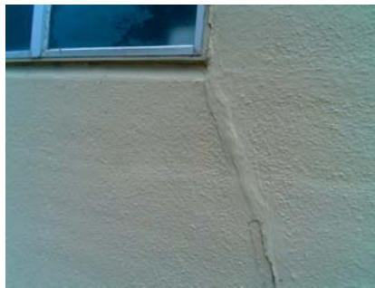
SW Primary Structural Type
