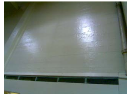
S Secondary Structural Type concrete form marks on inside walls.
