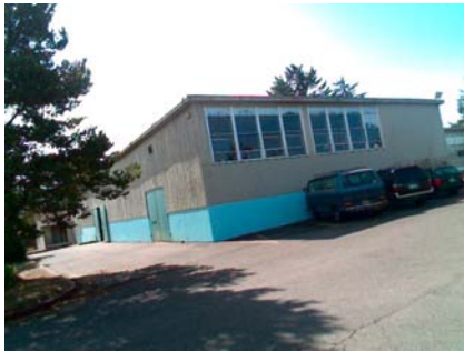
NE Elevation View
