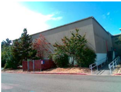
NE Elevation View
