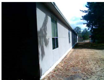
SW Elevation View
