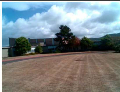
SW Elevation View
