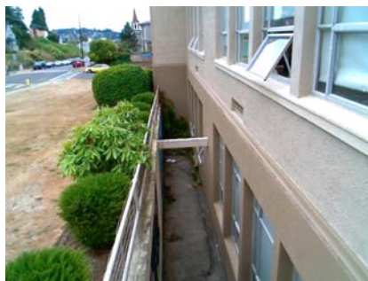
NE Pounding Potential retaining wall braced against bldg.
