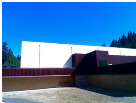
S Other white wall above is added mech screen, most likely stud framed. Not a part of pc gym framing.
