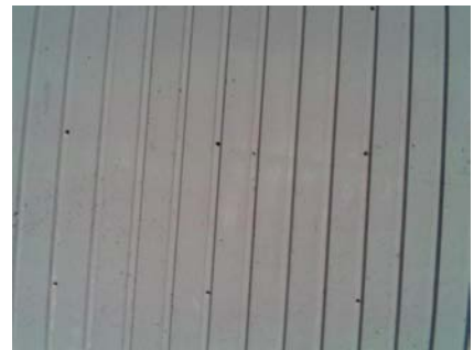
SW Primary Structural Type FORM TIE MARKS
